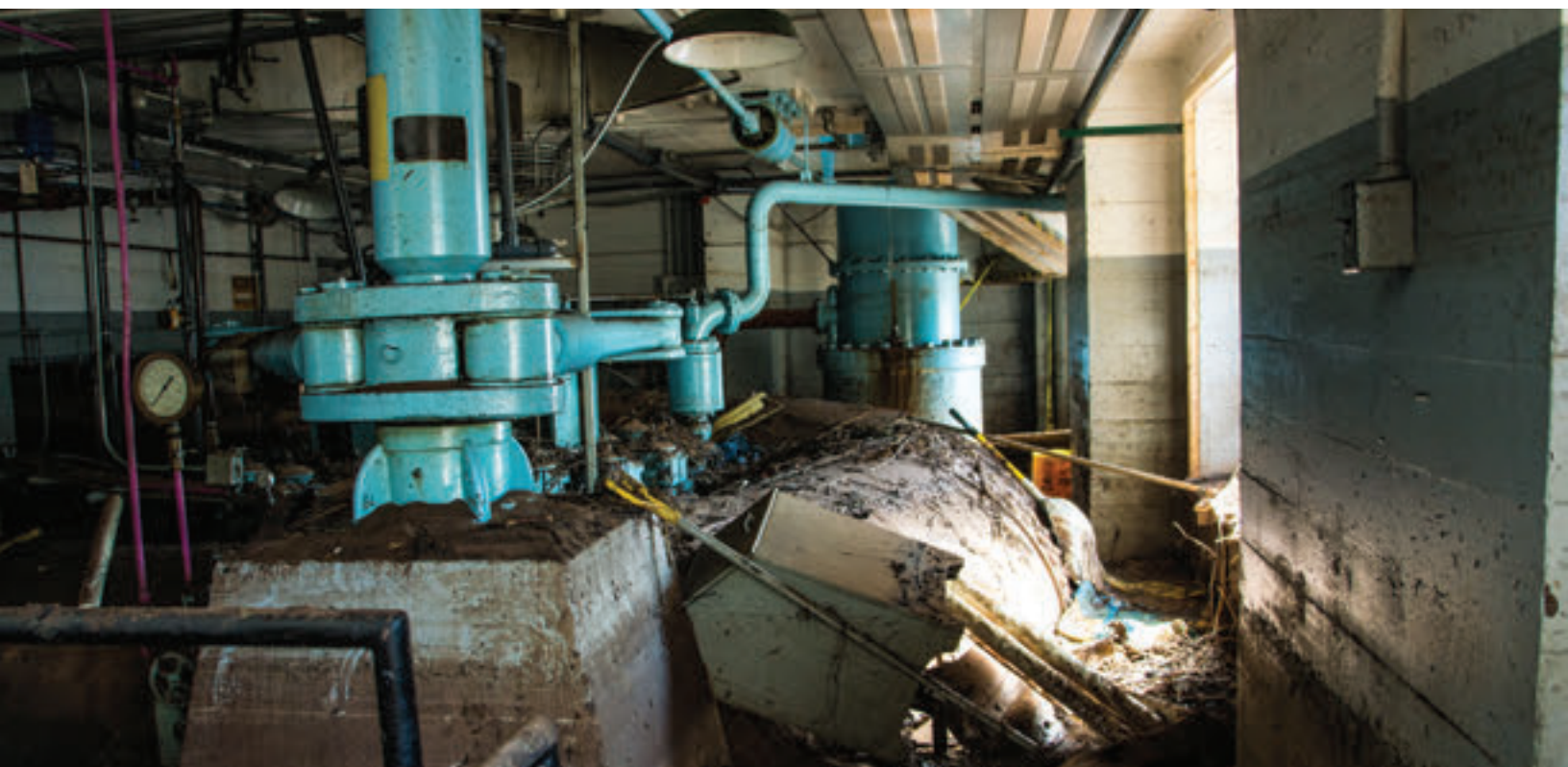
It took months to clean up the mud and debris left by flood waters that swamped the basement of the Thomson powerhouse.
