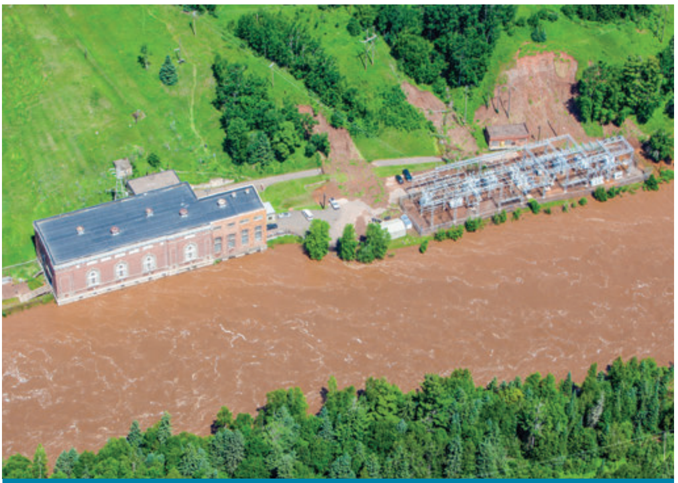
Mudslides washed out parts of the driveway to the Thomson powerhouse (left) and switch yard (right).
