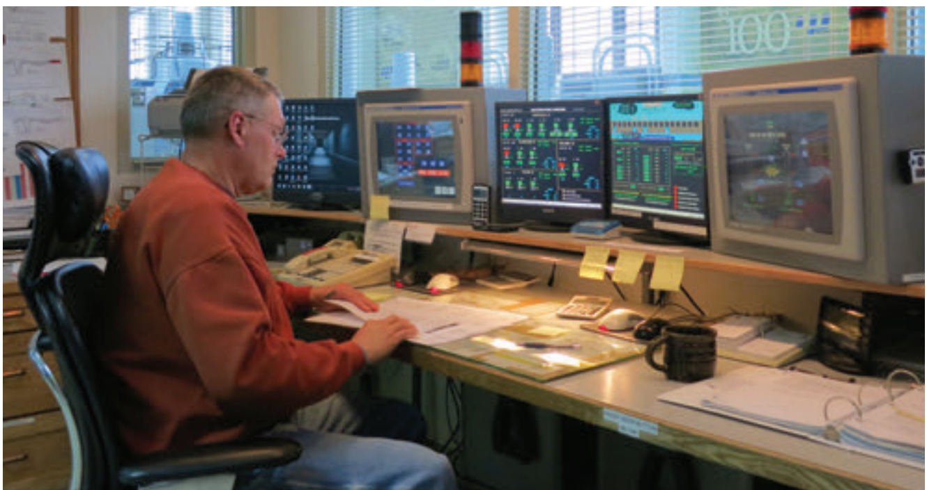
Roy Maki monitors flow levels from the control room at Thomson on a much quieter night several months later.
